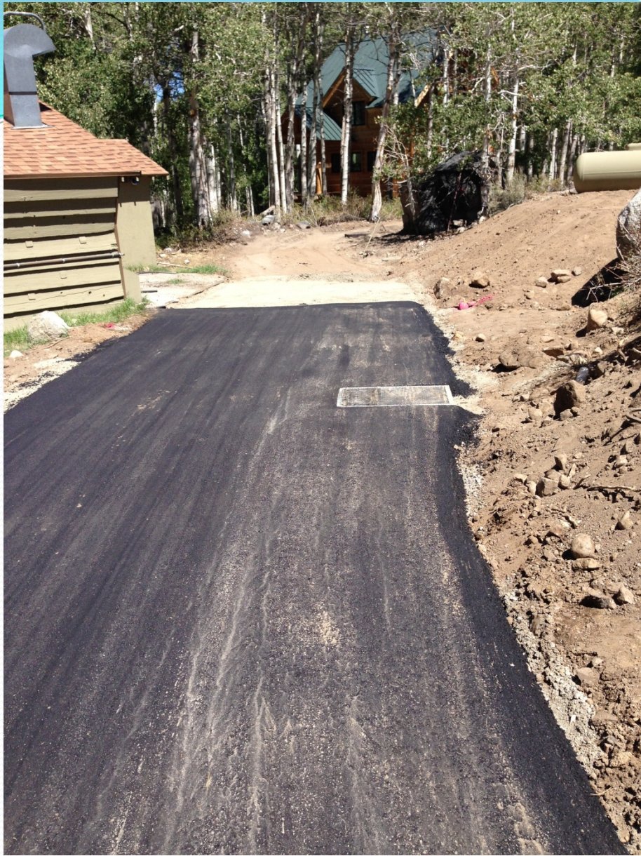
New pavement (Aspendell Mutual Water Company)
