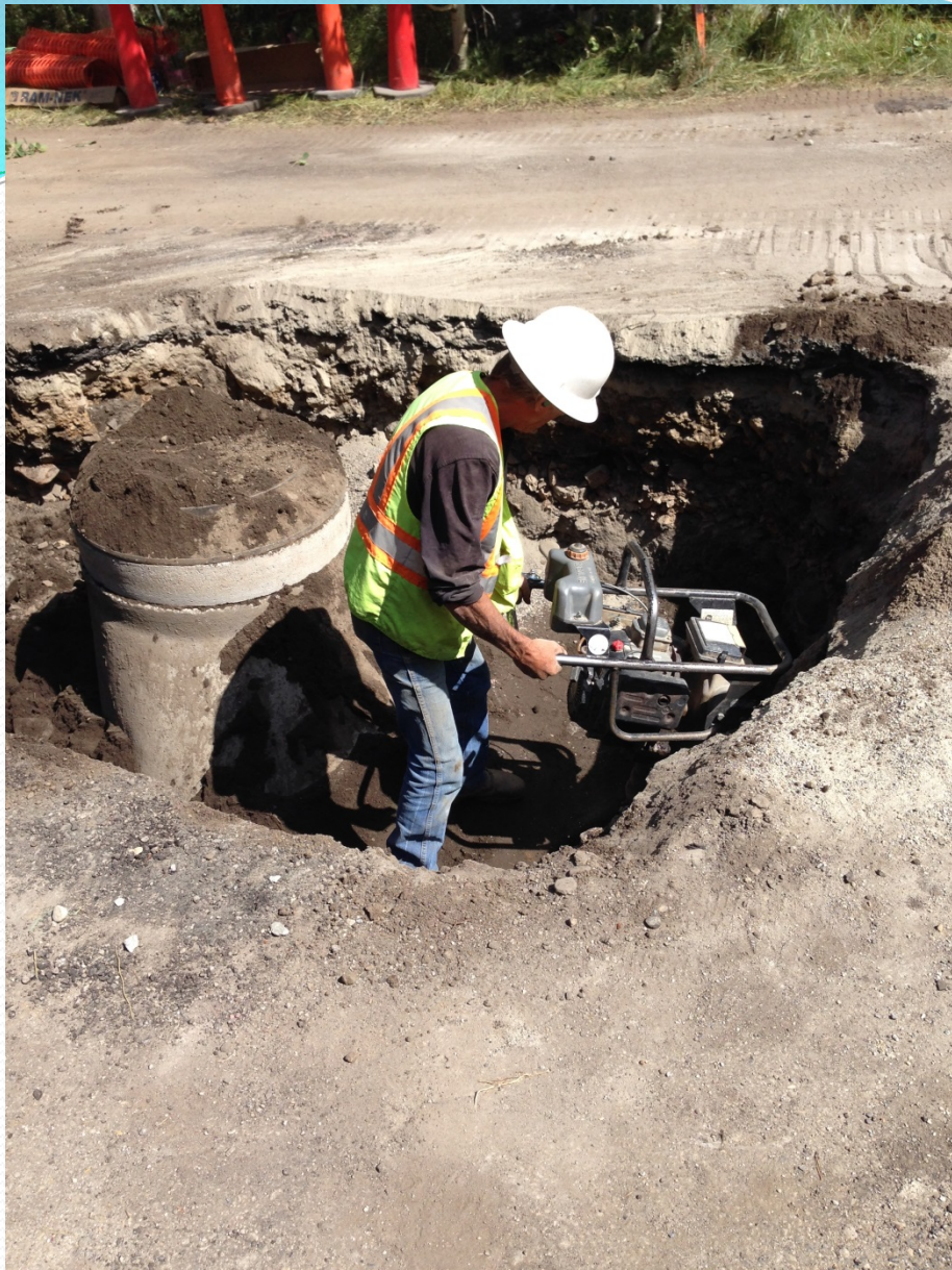
New sewer manhole; backfill compaction
