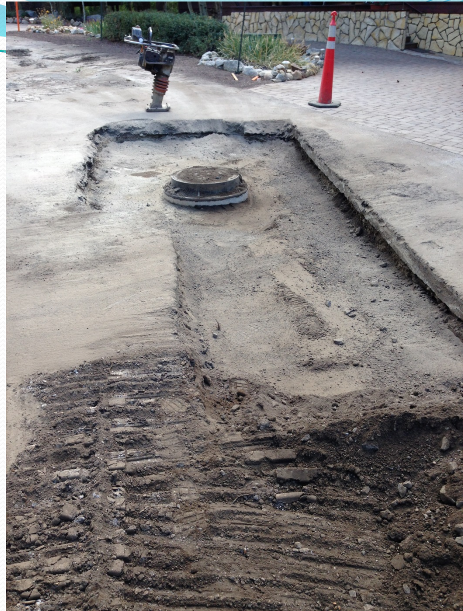
New sewer manhole; backfill compaction completed; ready for repaving
