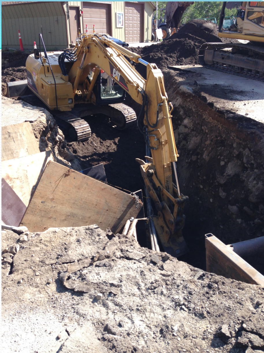
Backfilling new sewer line trench/excavation
