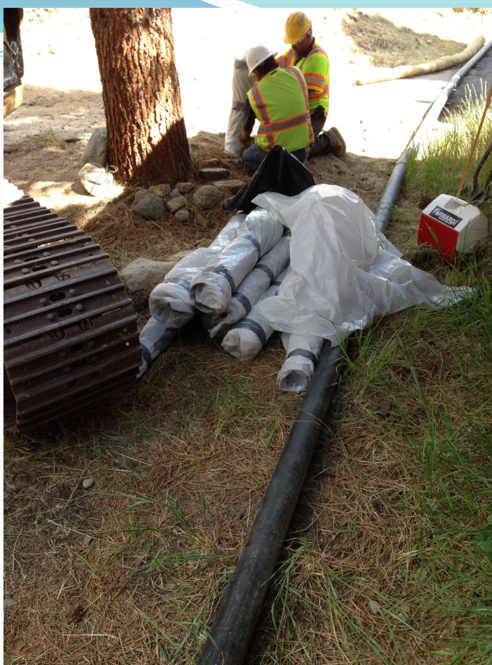
Preparing removed pieces of existing asbestos cement sewer pipe for disposal
