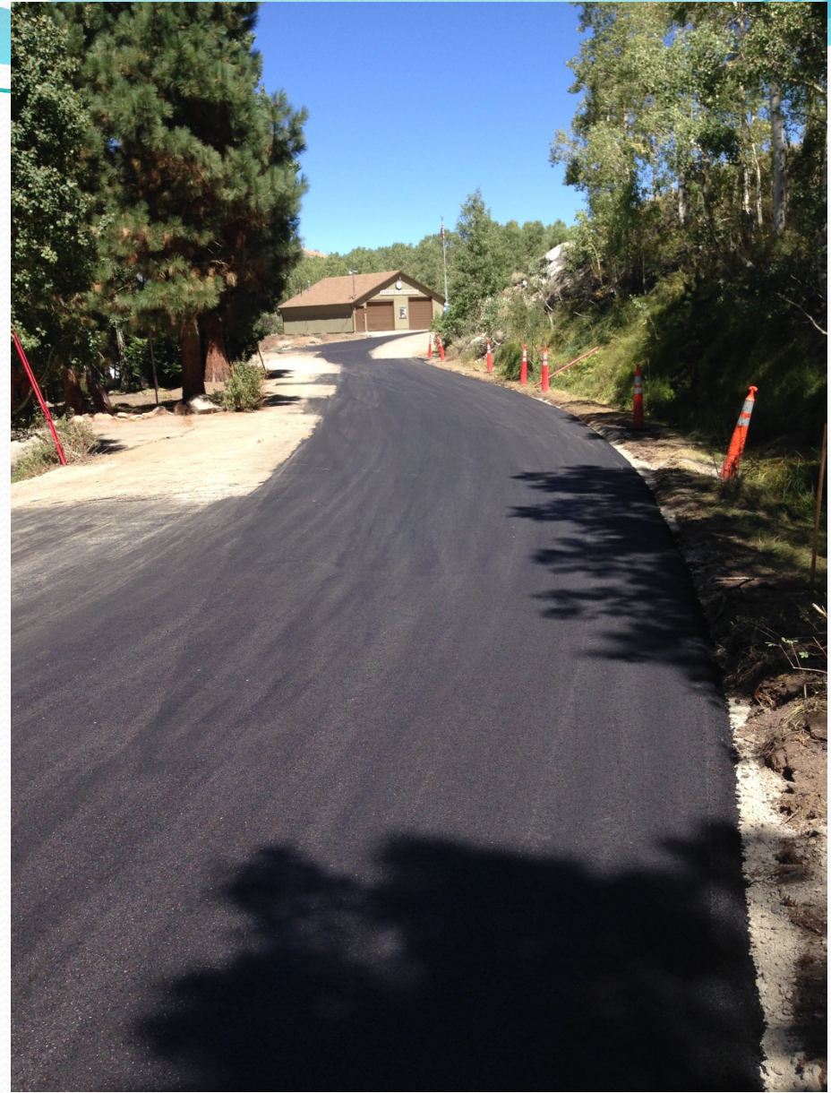
New pavement (Columbine Drive)
