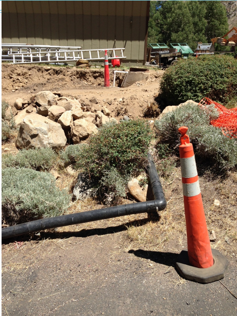
Temporary sewage bypass pipe (from one manhole to another)
