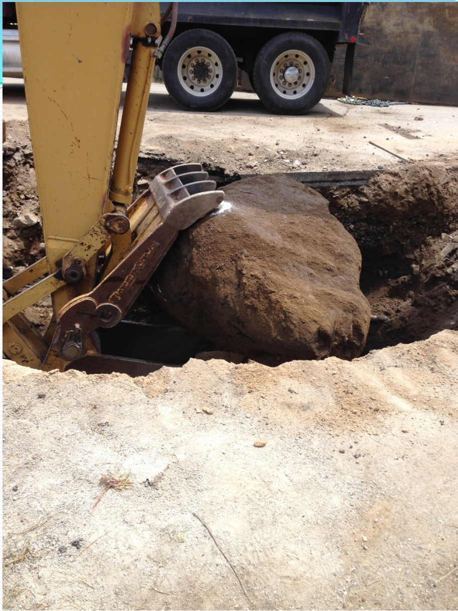
Removing large boulder from new sewer line trench
