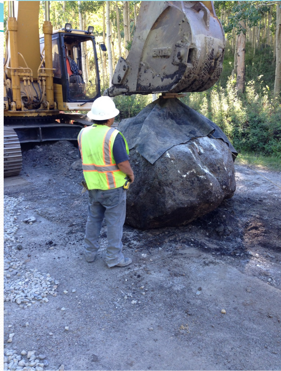
Large boulder prepared for blasting
