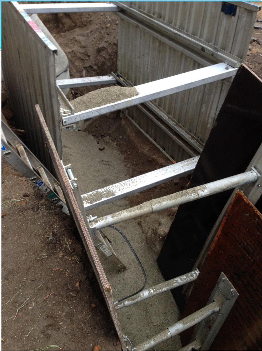
New sewer line trench/excavation with shoring and sand shading
