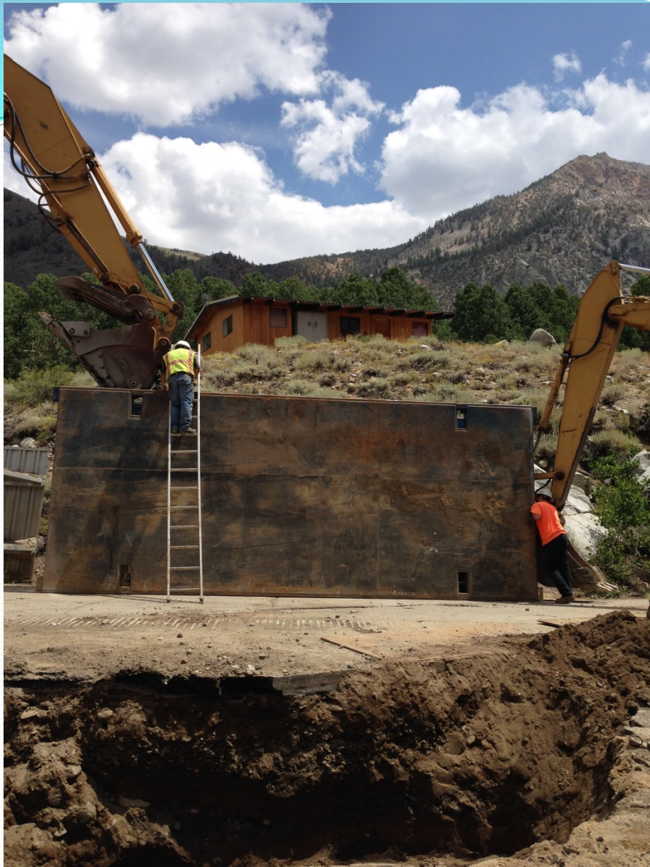
Preparing to lift trench box into deep sewer line trench/excavation
