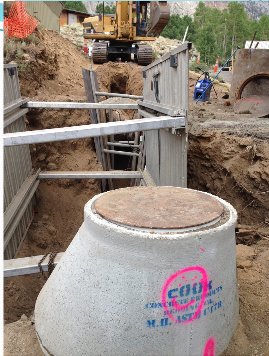
New sewer manhole and trench alignment/excavation with shoring
