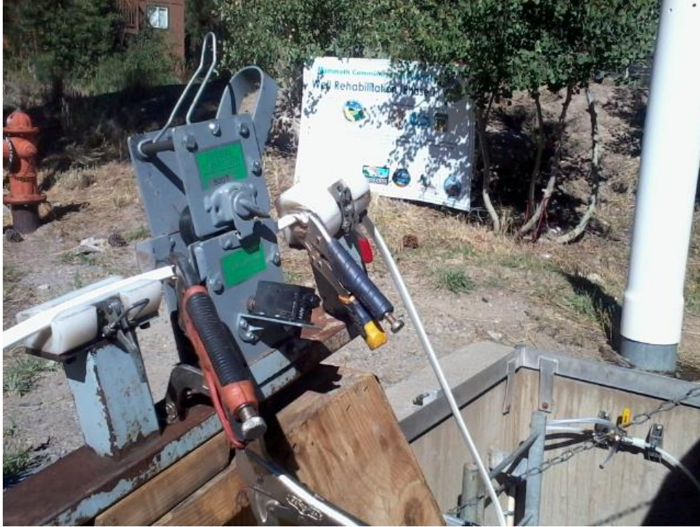
Above: Well-profiling instrumentation at sampling well.
