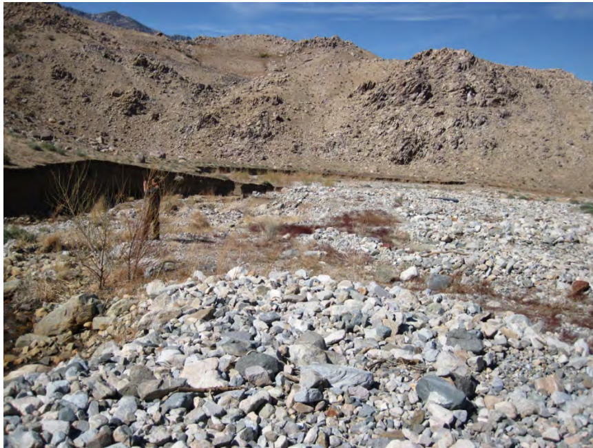
Figure 4 (Area where deposition has filled channel and forced flows against bank)
