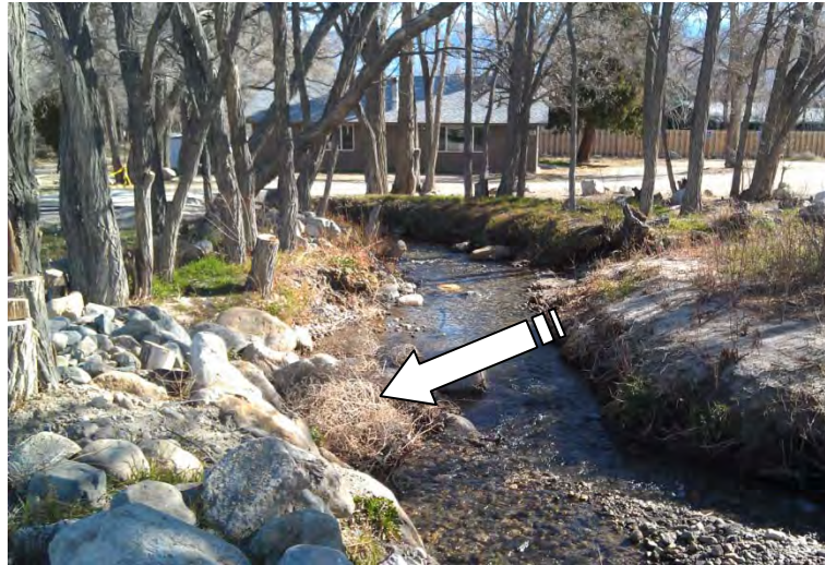
Figure 15 (Area for reshaping and fascine installation)
