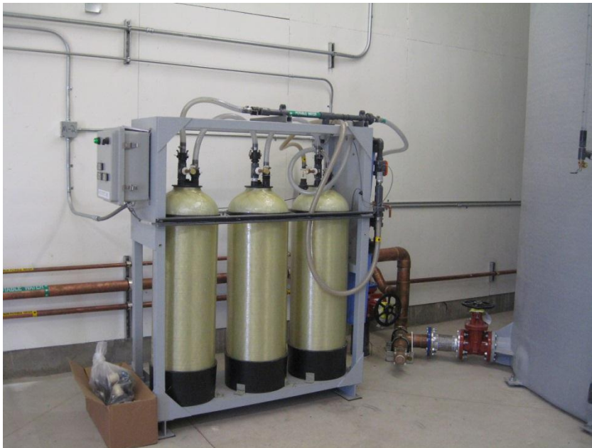
Ion exchange unit installed to remove uranium from well water.
