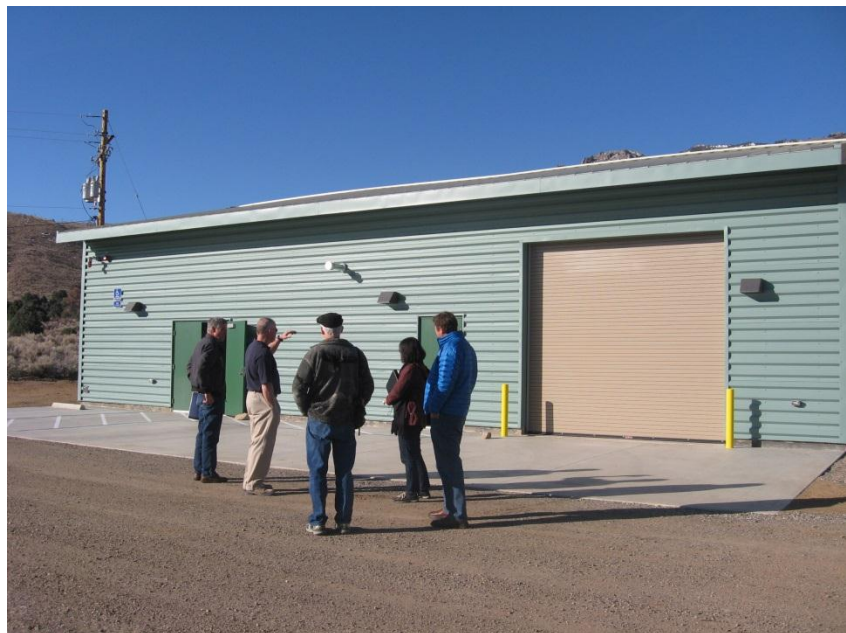
New building, housing ion exchange unit and storage tanks at Coleville High School.
