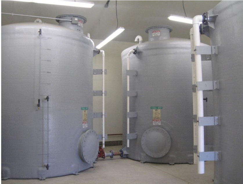
New storage tanks with a capacity of nearly 20,000 gallons of treated and untreated water.
