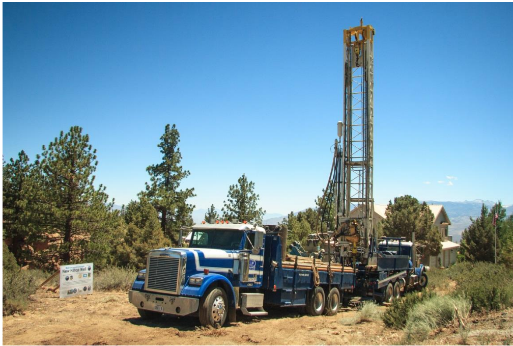
Drill rig at site of new well in Swall Meadows.
