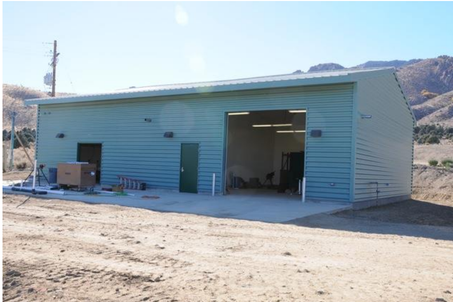
New building behind the Coleville High School (uphill from the football field) housing ion-exchange unit and three water tanks
